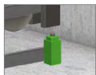
Switch for slack rope monitoring (governor rope)
