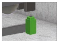
Switch for slack rope monitoring (governor rope)
