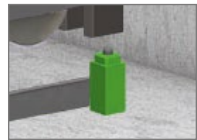
Switch for slack rope monitoring (governor rope)
