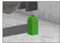
Switch for slack rope monitoring (governor rope)
